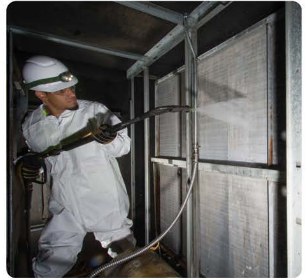
AQUIS Coil Restoration Process
